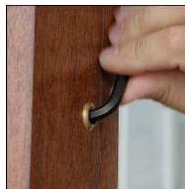
Screen/storm panel removal
